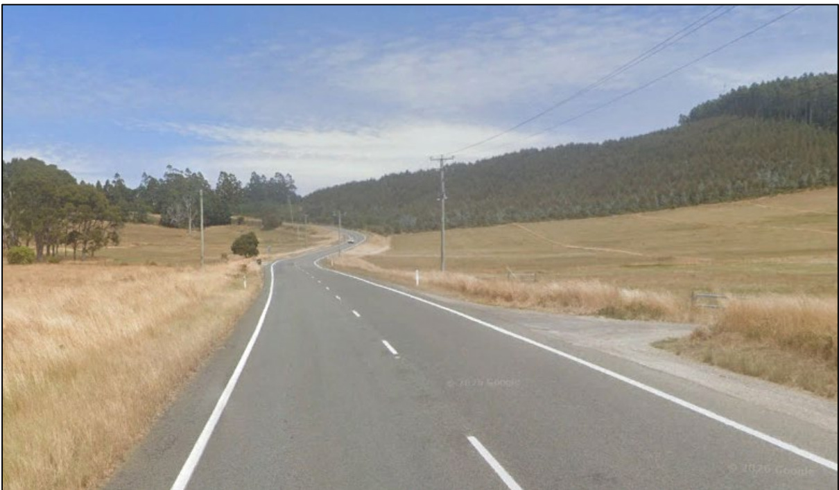
Figure 10: Existing vehicle access point onto Tasman Highway looking westward (Source: Google Maps).
