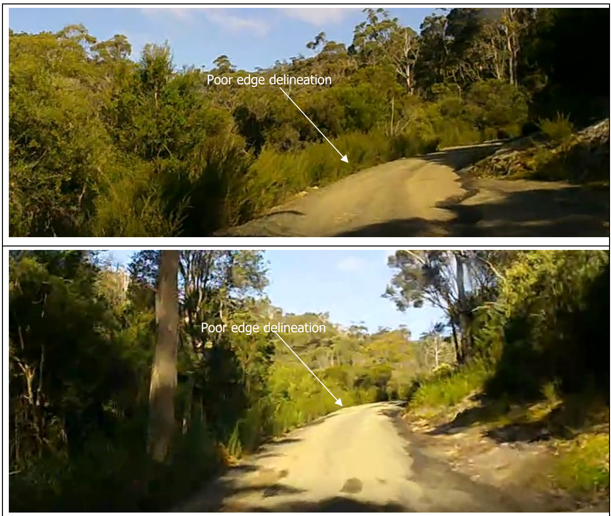
Figure 16 Poor Edge Delineation
