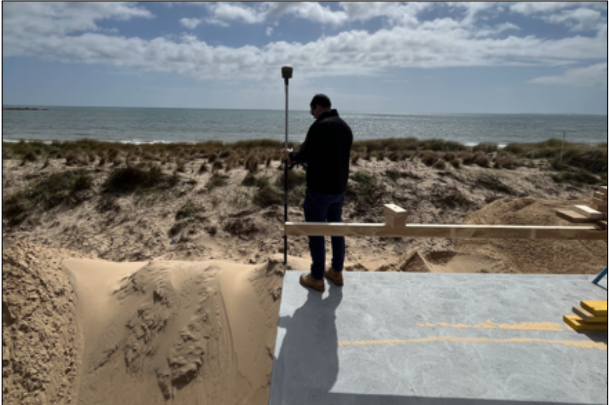
Photo 3 - photo illustrating the location of the survey point taken to confirm the location of the north-western most corner of the currently under construction Unit 08.
