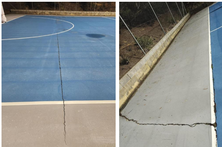
Image 2 & 3: Bridport – Existing Court 1
