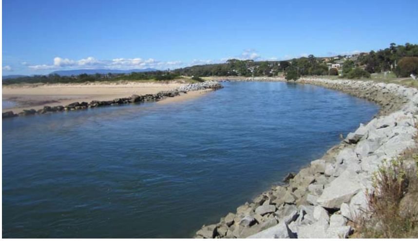
engineered sea wall and inlet channel
