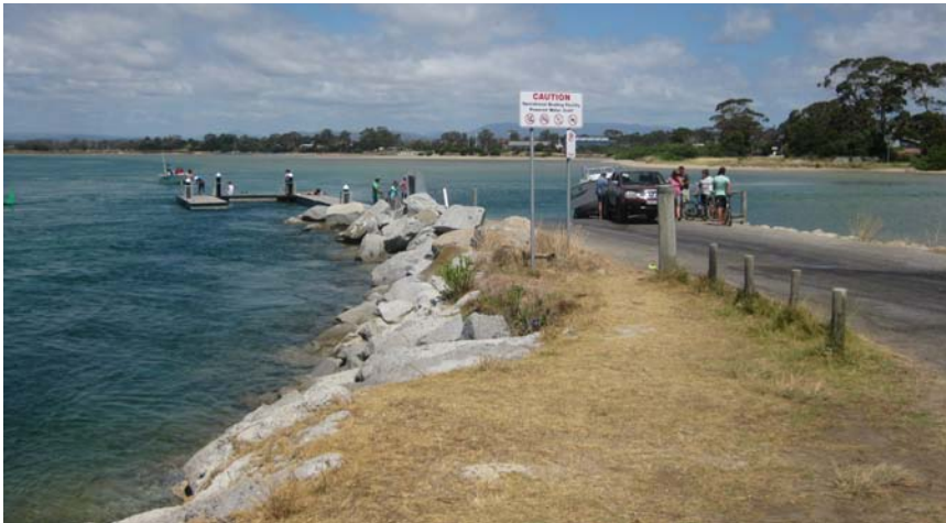
boat ramp, pontoons & rock wall along inlet
