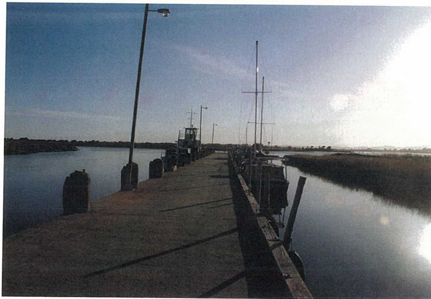
Figure 29: The main wharf at Bridport
