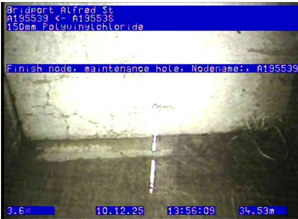
A195272_a0c5ca9f-77aa-401f-8c61-2017e295f54e_20251210_135625_014.jpg, 00:04:56, 34.53 Finish node, maintenance hole, Nodename:, A195539
