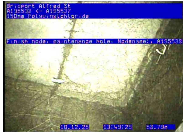
A195273_361c28c9-eb3a-48d2-8170-3442ba8b9800_20251210_134944_239.jpg, 00:08:13, 58.79 Finish node, maintenance hole, Nodename:, A195538
